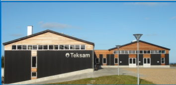
Teksam Headquarters in Denmark
